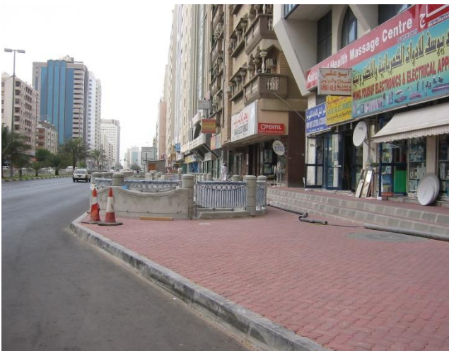
due to the limited space between high-rise buildings and the street, there was no alternative to our tunnel construction
