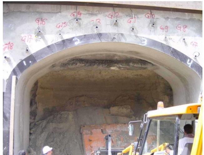
after grouting, excavation with a JCB
