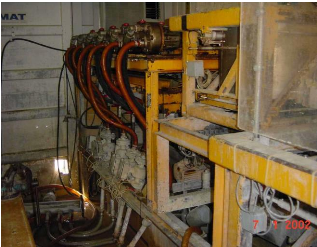
Pump container for grouting the injection pipes
