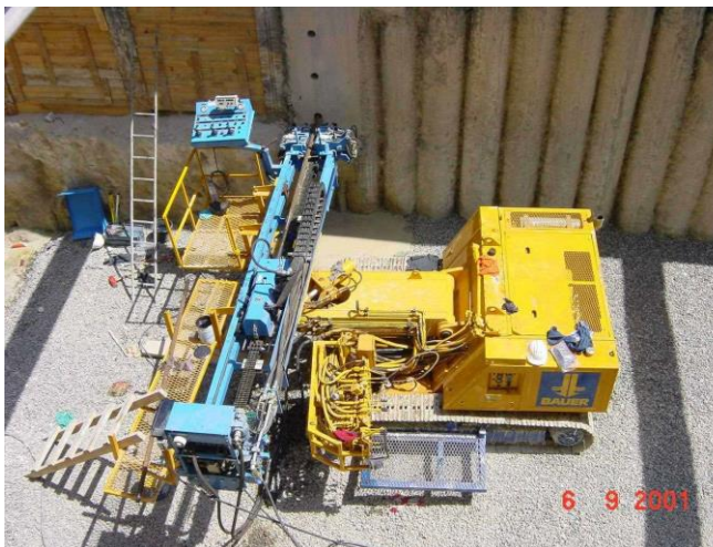
for the tunnels, special self-built drilling rig
