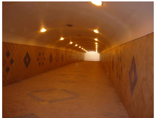
a completed tunnel
