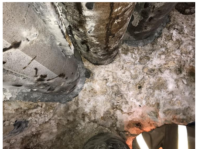
only 20 mm tolerance in the pipe arch, annulus was grouted
