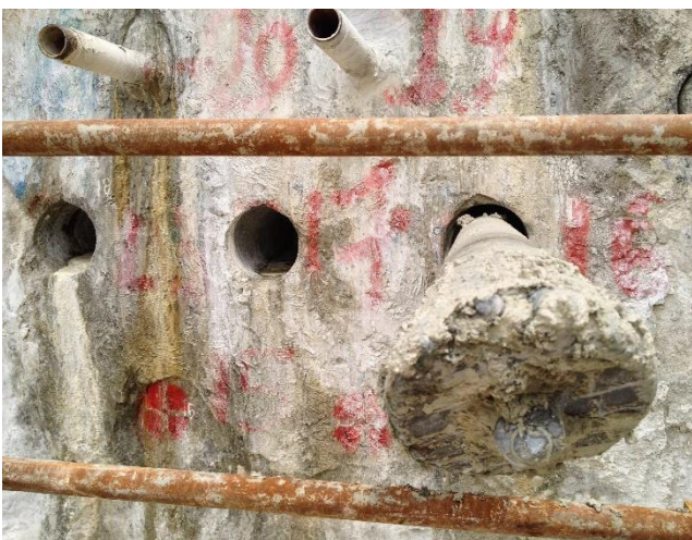
All boreholes require 100% drilling out of the pre-cored holes in the bored pile wall
