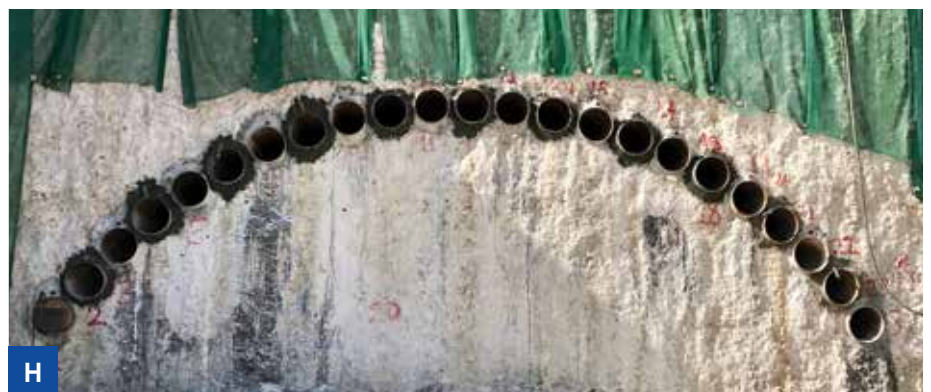
F: The FS508 with DHT hammer. G: The BM600LS with the FS508 and the pipe arch. H: The pipe arch tunnel 3. Starting shaft. I: The pipe arch tunnel 3. Receiving shaft. J: The metro access tunnel after all construction works have been completed.
