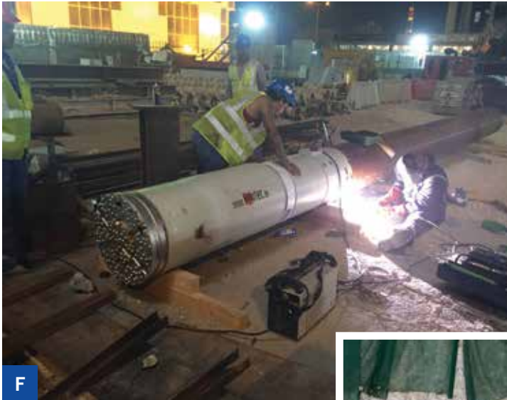
F: The FS508 with DHT hammer. G: The BM600LS with the FS508 and the pipe arch. H: The pipe arch tunnel 3. Starting shaft. I: The pipe arch tunnel 3. Receiving shaft. J: The metro access tunnel after all construction works have been completed.
